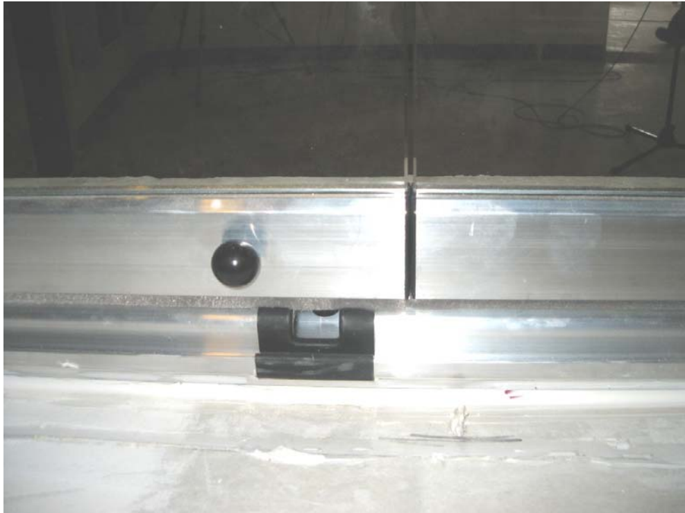
Fig. 3: View Transmission Room, Measurement 1, Detail
